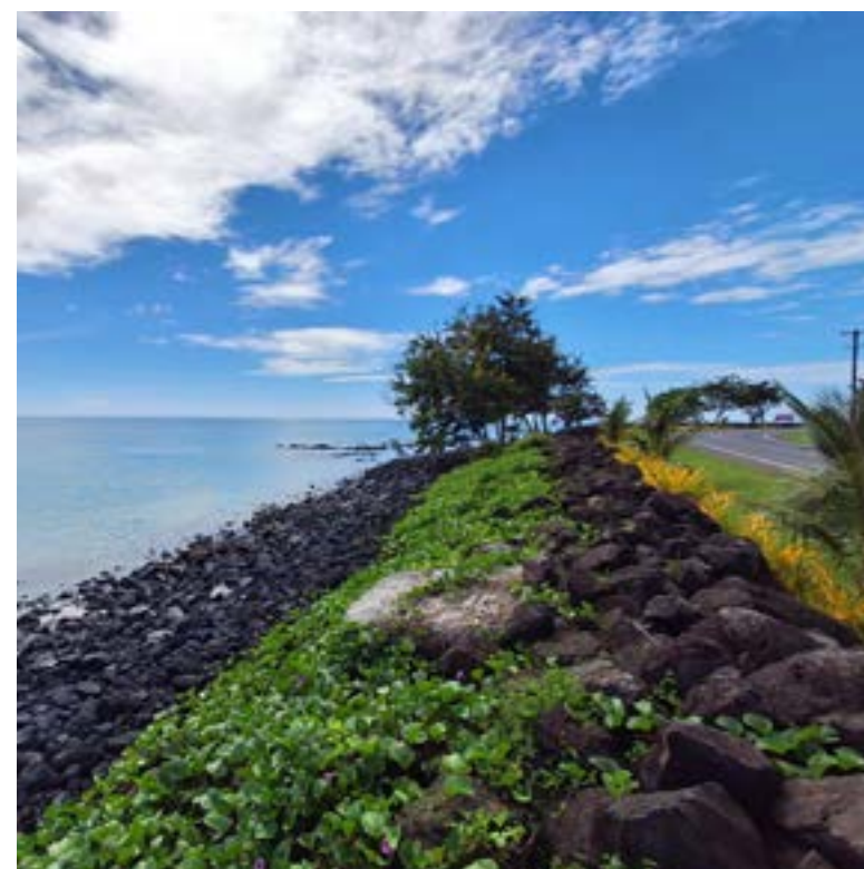
Coastal strengthening, Upolo Island, Samoa. Photo by Dao Polsiri.
