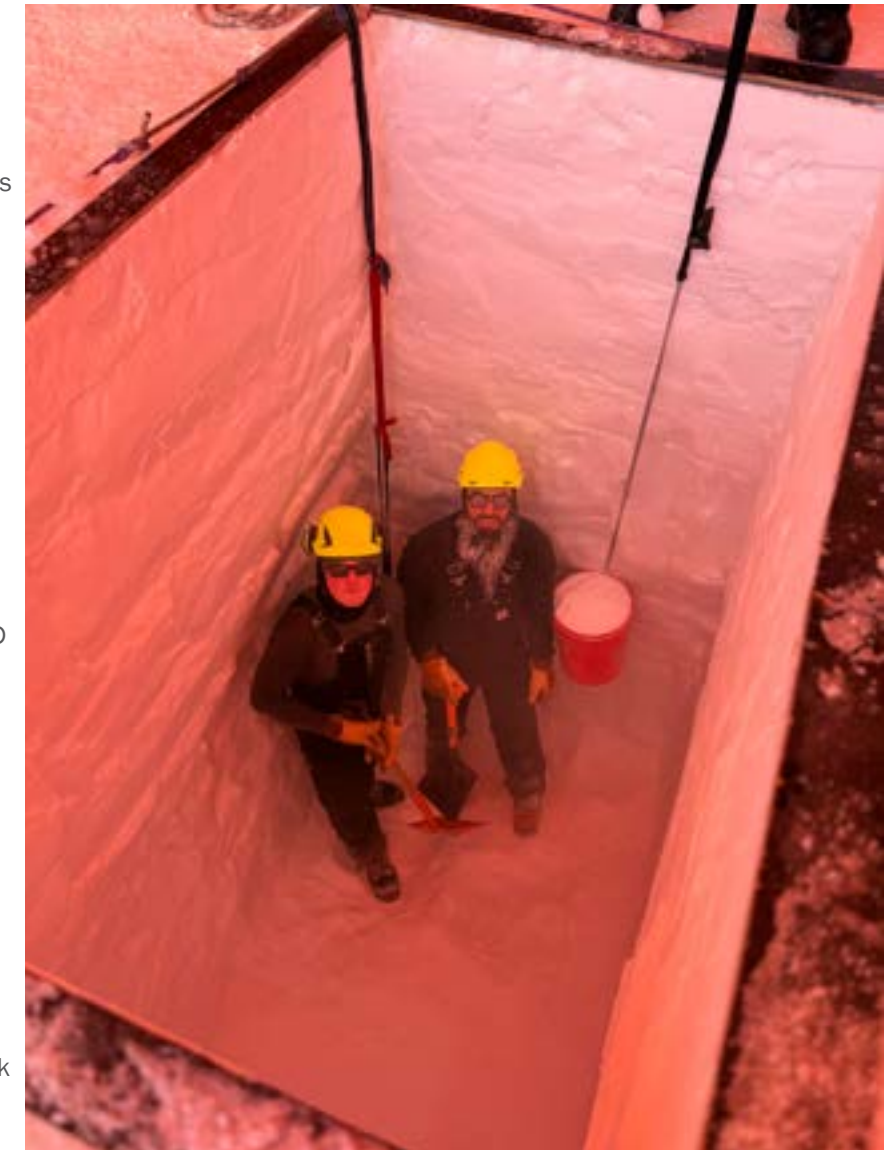
James MacPhail (left) and driller Tim McPhee digging the AIDD cellar, setting up for drilling operations at Kamb Ice Stream. The cellar provides clearance under the drill rig floor to enable installation of long items and to keep sea riser support equipment clear. Photo by Jane Chewings.
